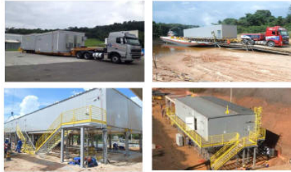
Figure 85 Modular electrical substation – transport and assembly
