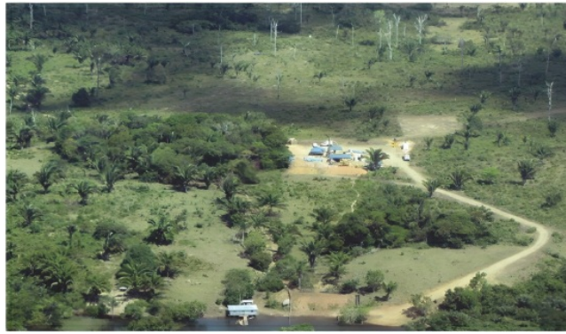
Figure 16 View of drill site location for the drill holes PBAT 15-43 and PBAT 15-43 A (SRK, 2016, /50/)
