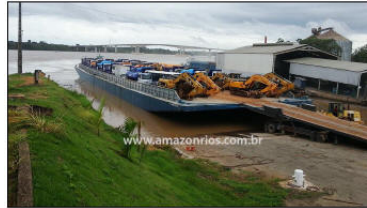
Figure 96 General cargo raft and concrete ramp with adjustable metallic ramp (WorleyParsons and PdB, 2022, /59/)
