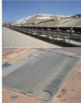
Figure 128 Photos of views with typical dry stacking installation planned for the formation of the tailings piles (Emerson, 2021, /13/)
