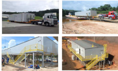
Figure 85 Modular electrical substation – transport and assembly
